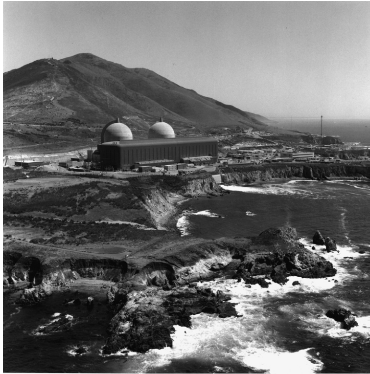
FIGURE 12.9 A nuclear power plant, Diablo Canyon, on the California coast (Courtesy Pacific Gas & Electric Company).
